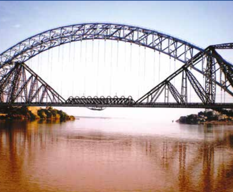
Lansdowne Bridge, Rohri
